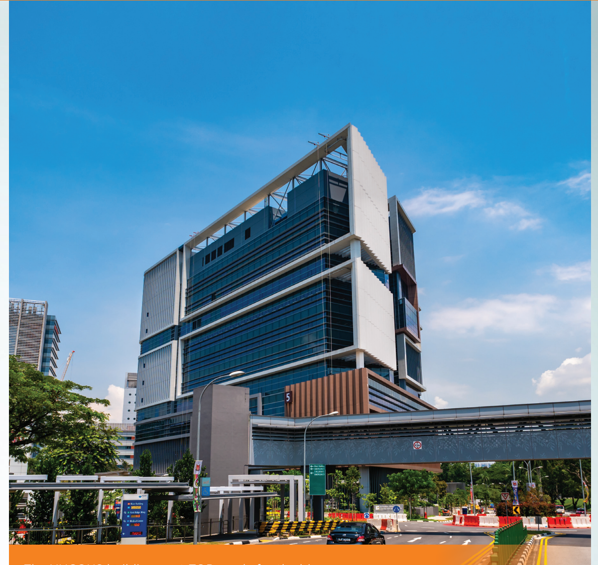
The NUCOHS building post-TOP, ready for the big move.
